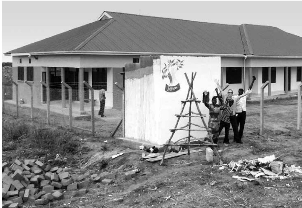
Construction on the Yotkom Medical Centre.
